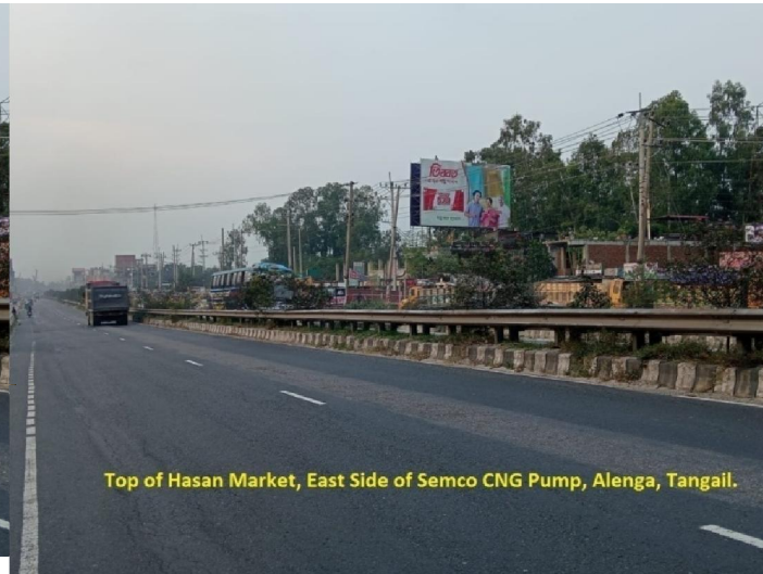
Top of Hasan Market, East Side of Semco CNG Pump, Alenga, Tangail.
